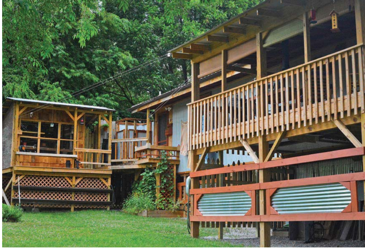
The McGarvey home, an 830-square foot green built structure in Candler. (above) James and Cilla McGarvey. (below) Garret K Woodward photos
